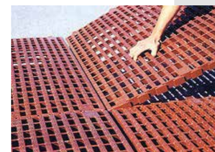
Detail of grid's assembly
